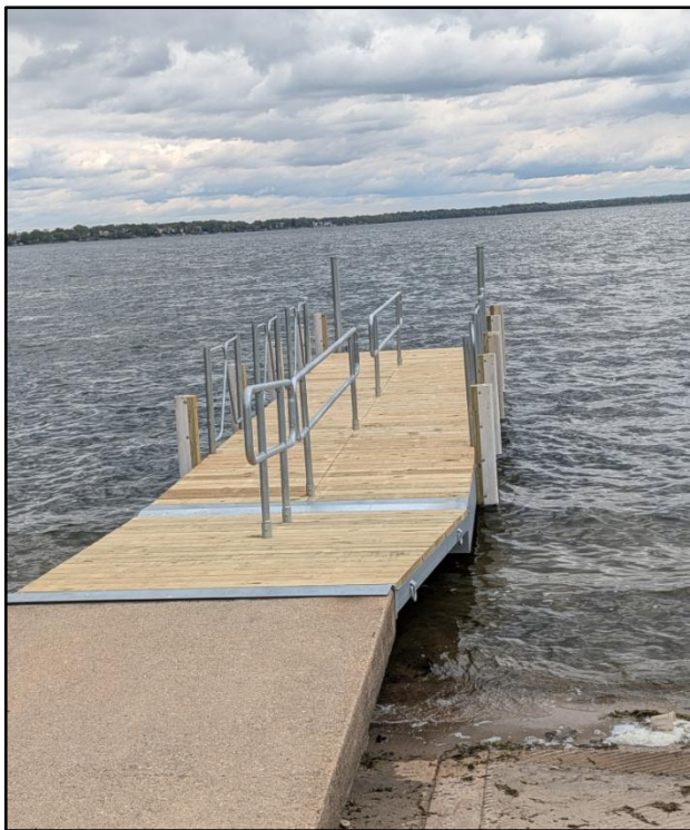
New dock installed at the Olin Park boat launch
